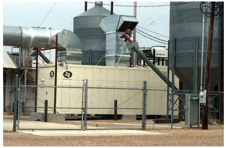
2G Patruus 280kWe unit (left) and 500kWe Agenitor Twinpack (right) at O'Hair's manufacturing facility in Lubbock, Texas
