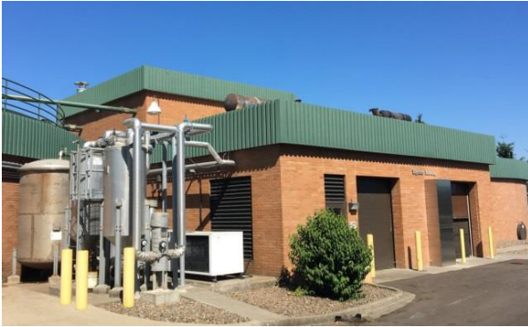
Gresham Wastewater Treatment Plant
