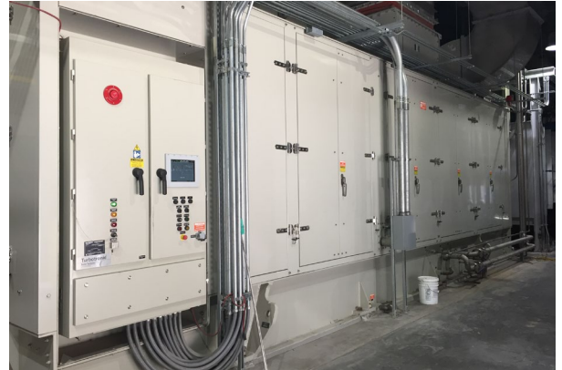
7 MW CHP Gas Combustion Turbine at Vanderbilt
