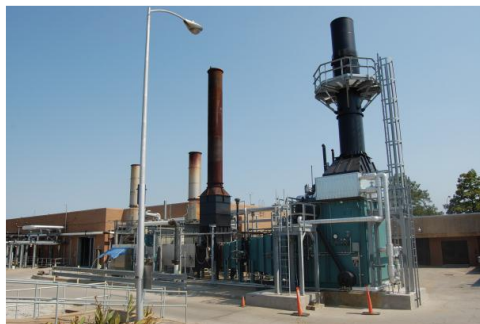
Biogas Turbine (left) and Heat Recovery Steam Generator & Duct Burner (right)
