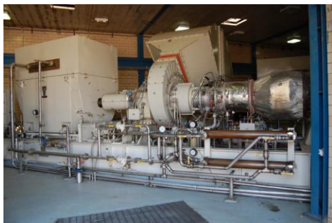
Biogas Turbine (left) and Heat Recovery Steam Generator & Duct Burner (right)
