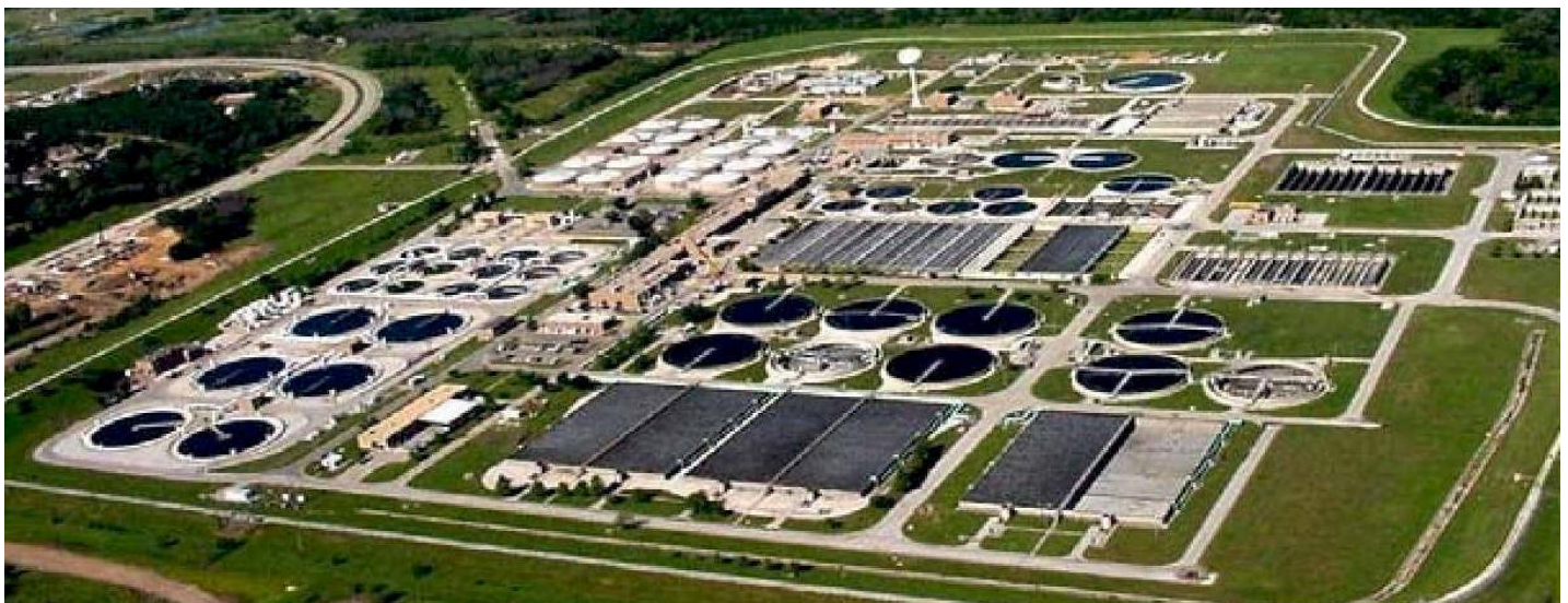
Village Creek Water Reclamation Facility, Fort Worth Water Department
