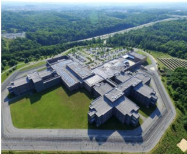
The Montgomery County Correctional Facility 200 kW CHP and 2.8 MW PV microgrid
