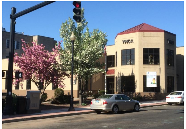
The Meridian YMCA in Connecticut uses a PACE-financed 60 kW CHP system that provides electricity and hot water.
