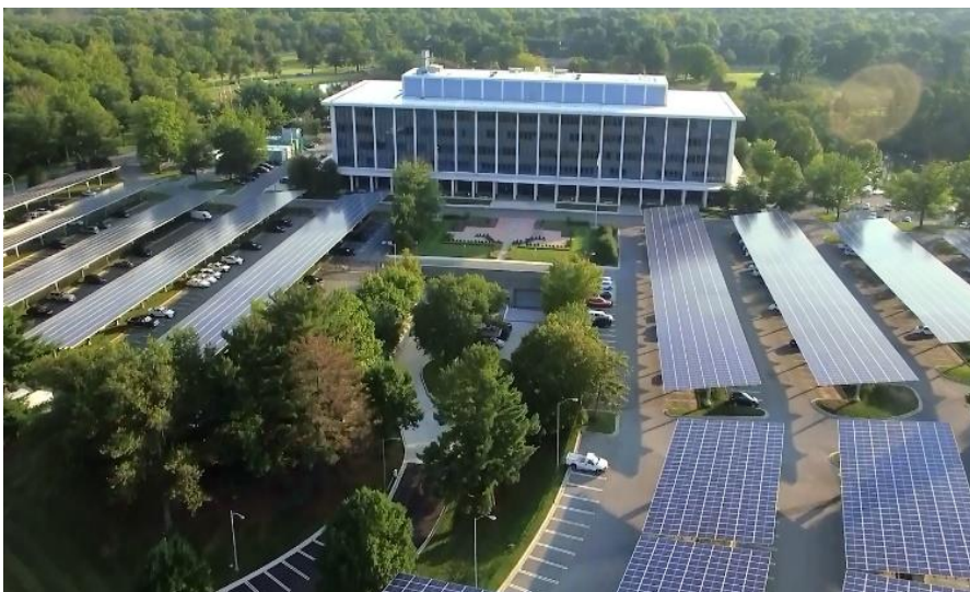
Montgomery County Public Safety Headquarters Microgrid (1,014 kW CHP System and 2 MW PV)
