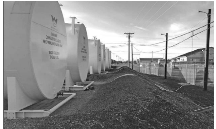
AVEC built a new 360,000-gallon bulk fuel storage facility.
