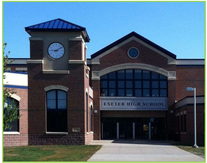
The Exeter School District is supplied by a 65 kW microturbine and 100 kW ground-mounted solar PV.
