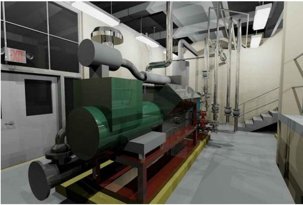
**At the Downers Grove Sanitary District, CHP units can produce up to 660 kW of electricity. Utilized alongside major energy efficiency improvements throughout the facility, the CHP system assists the sanitary district in its journey to net-zero energy status.**
