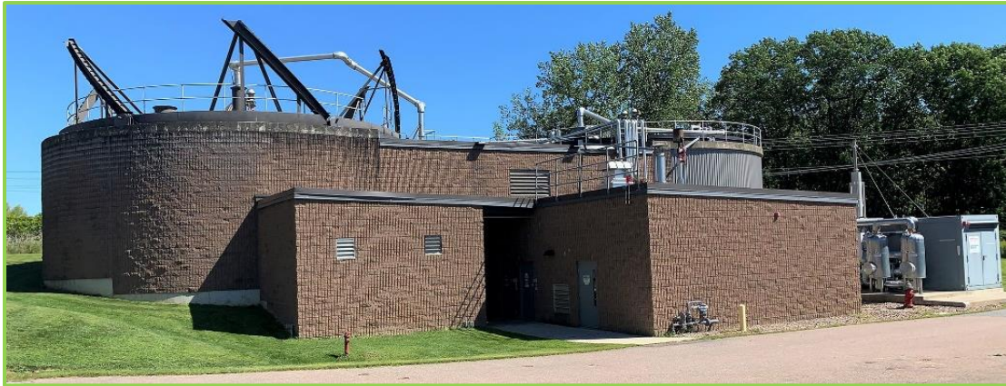
Anaerobic digester (left) with the new CHP system (right)
