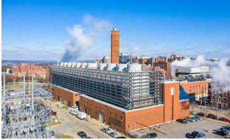
New Central Utility Plant (includes the 47 MW CHP system)
