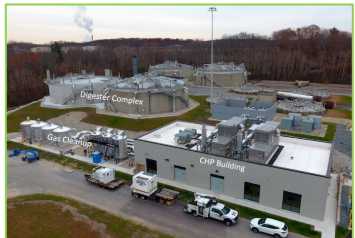
GLSD CHP Building and Gas Process
