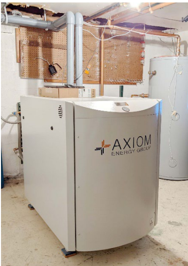
Axiom 4.4 kW Micro CHP System Source: Axiom Energy Group
